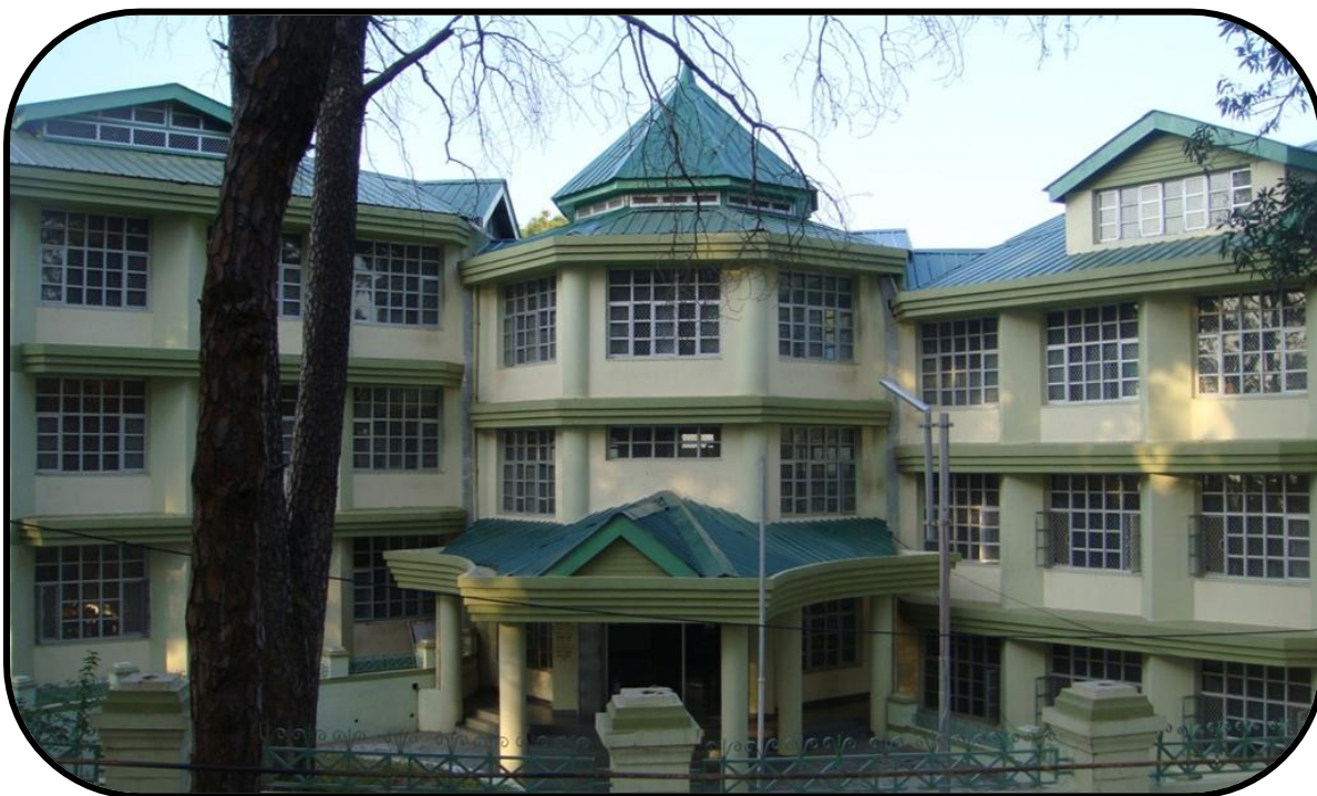
District Court Complex – Sirmour at Nahan
